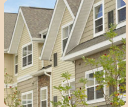
The Greens at Rolling Road
